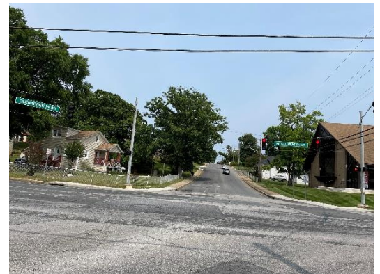
Removal and repair concrete sidewalks, curb and gutters on Glenarden Pkwy. from Brightseat Road to Jeff Road
